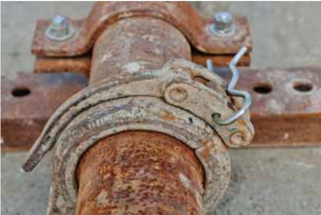
Concrete pipe clamps with safety pins
