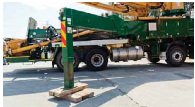
A concrete pump truck with its outriggers extended and pigstyed.
